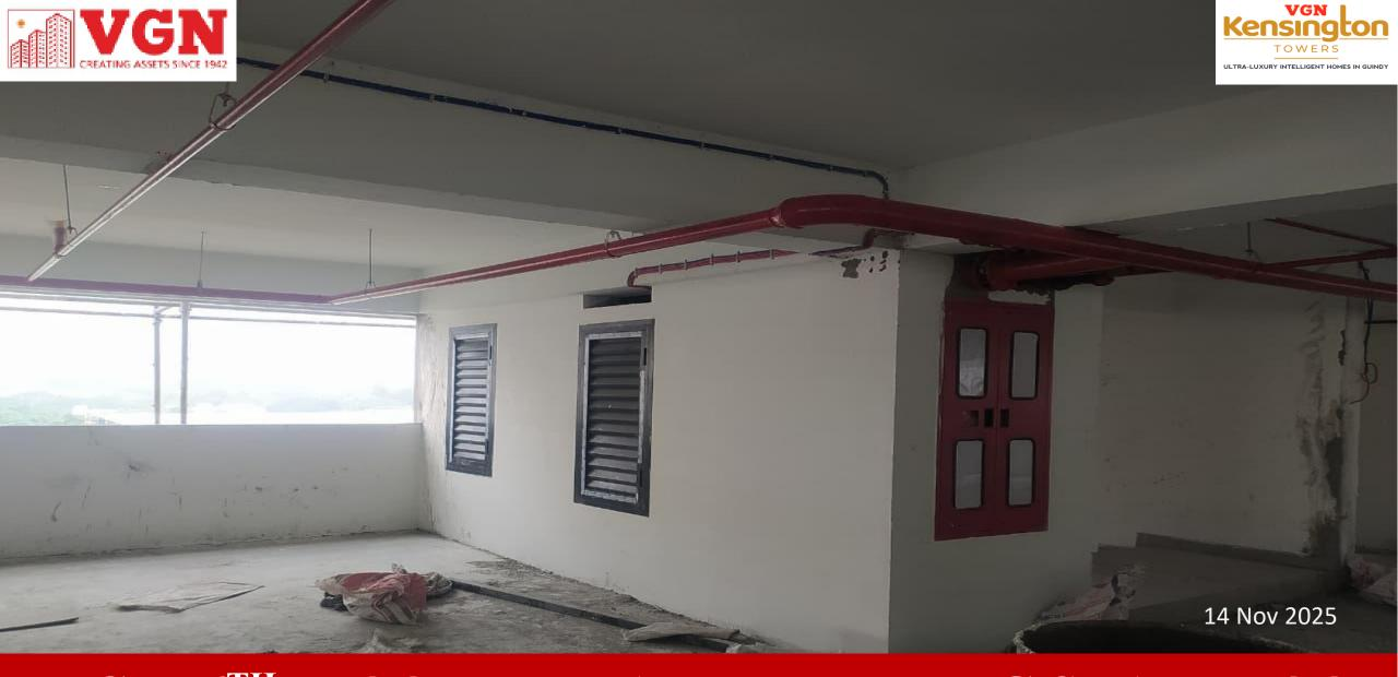
MLCP - 6<sup>TH</sup> FLOOR FIRE AND PLUMBING SHAFT DOOR FIXING WORK HAS BEEN COMPLETED
