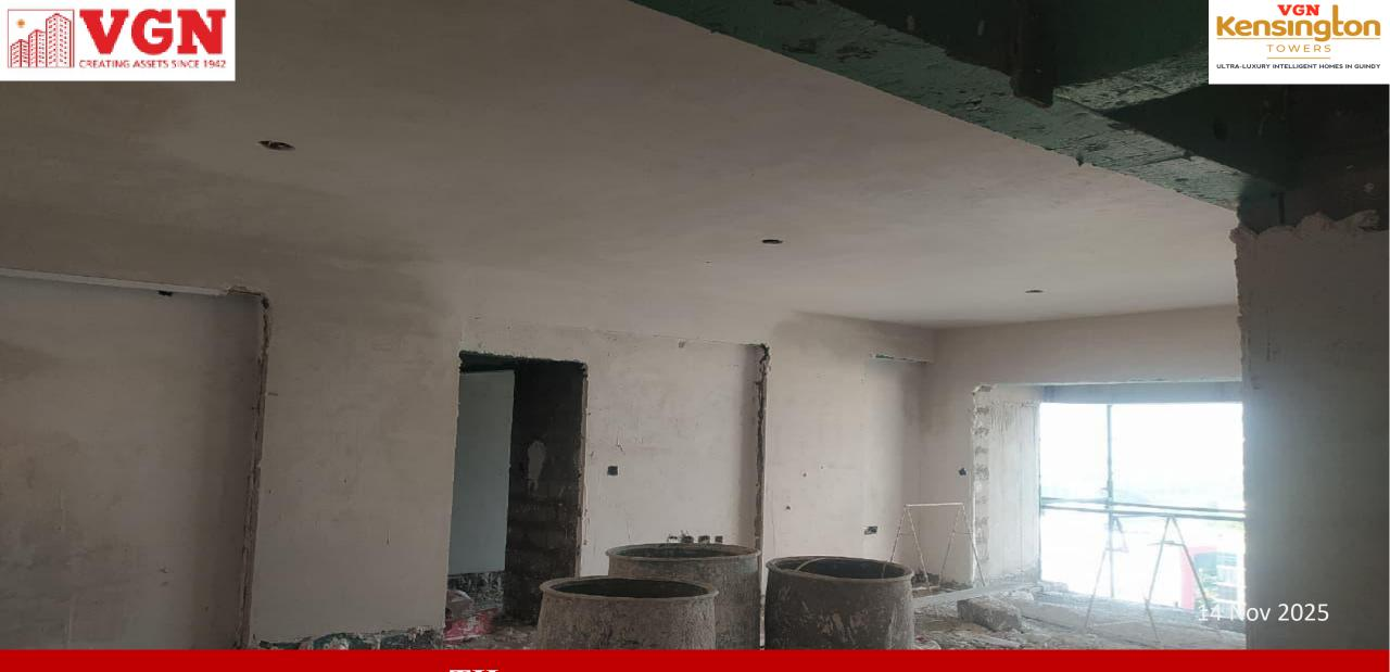
C4 BLOCK- 12<sup>TH</sup> FLOOR GYPSUM PLASTERING WORK IN PROGRESS
