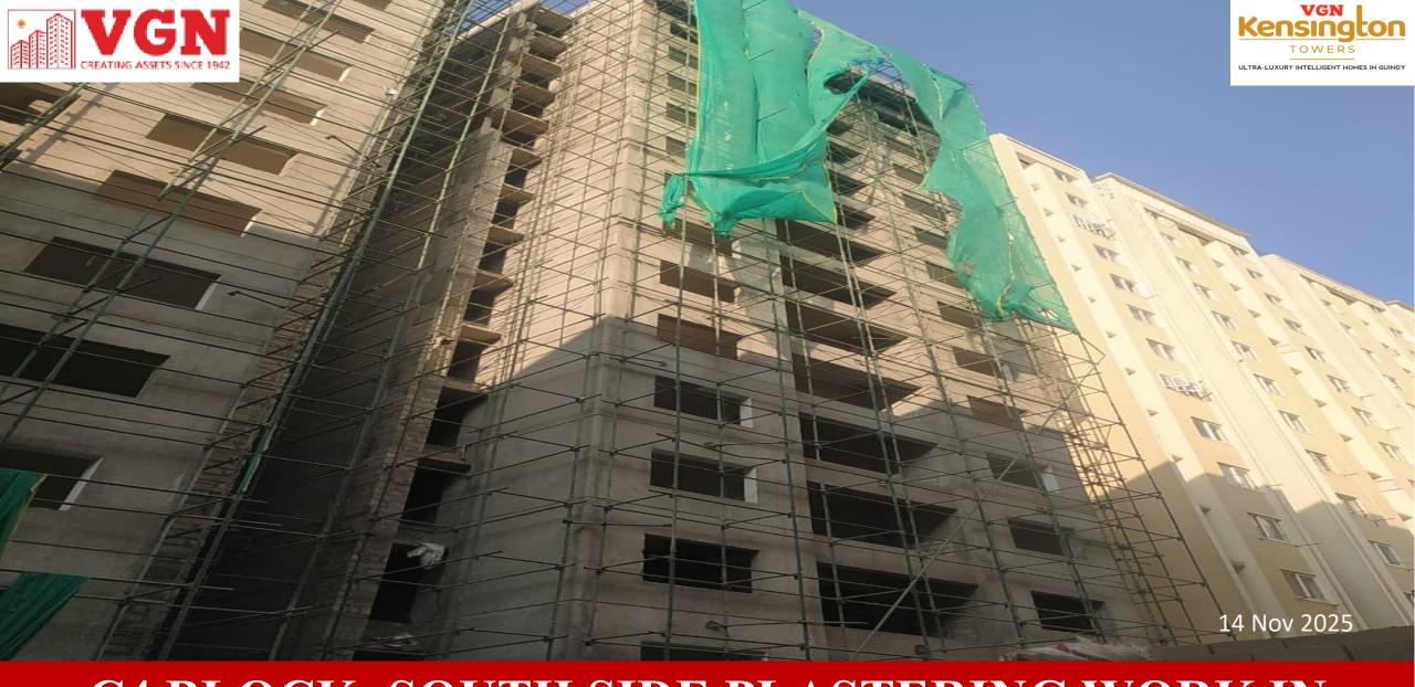
C4 BLOCK- SOUTH SIDE PLASTERING WORK IN PROGRESS
