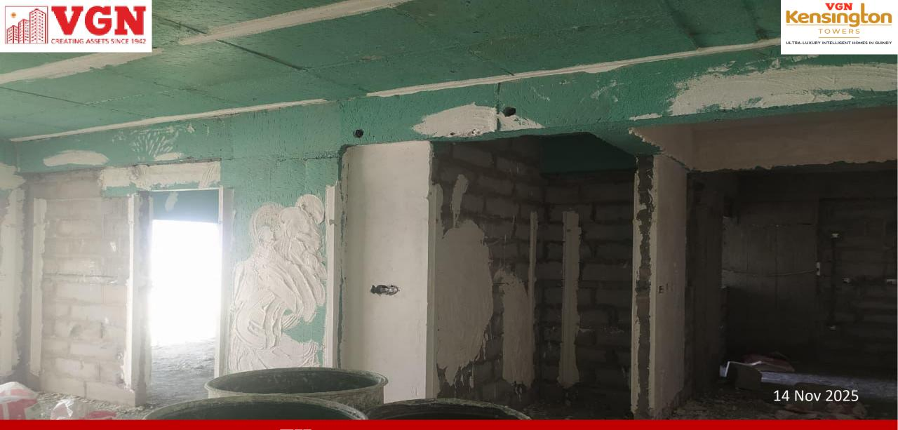
C3 BLOCK- 12<sup>TH</sup> FLOOR GYPSUM PLASTERING WORK IN PROGRESS
